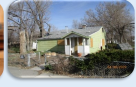
Increased Code Violations affecting Neighborhood Safety
