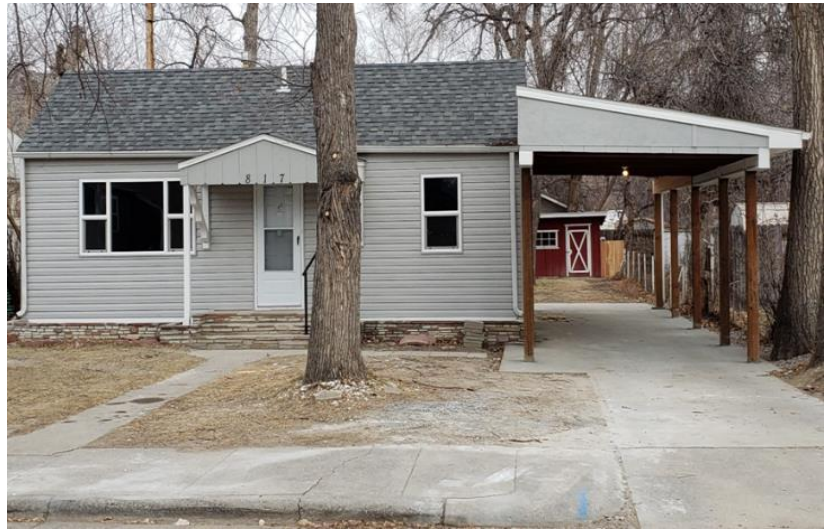
North Park rehabilitation project
